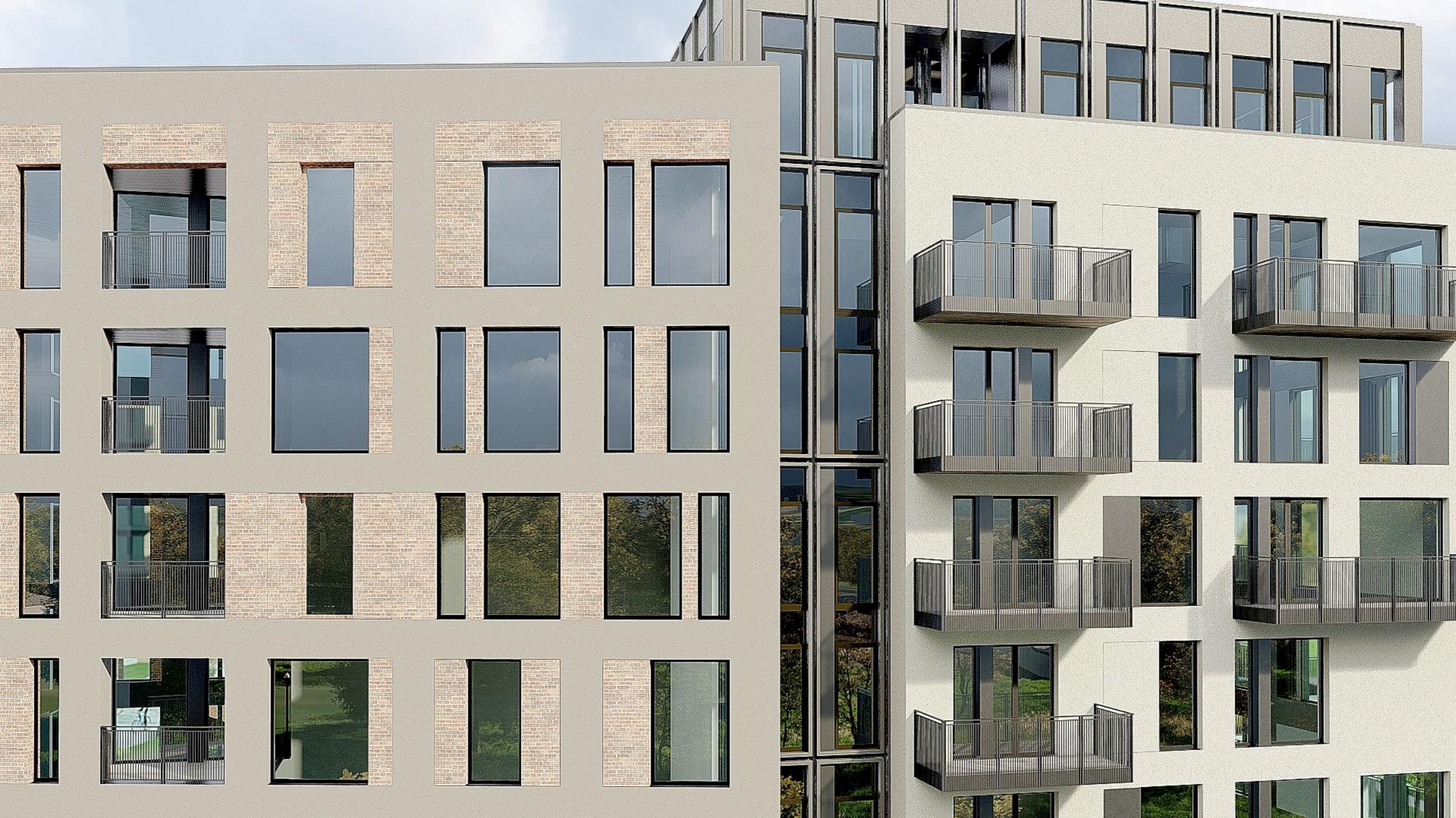
MATERIALITY: BUILDING D –EAST FAÇADE
